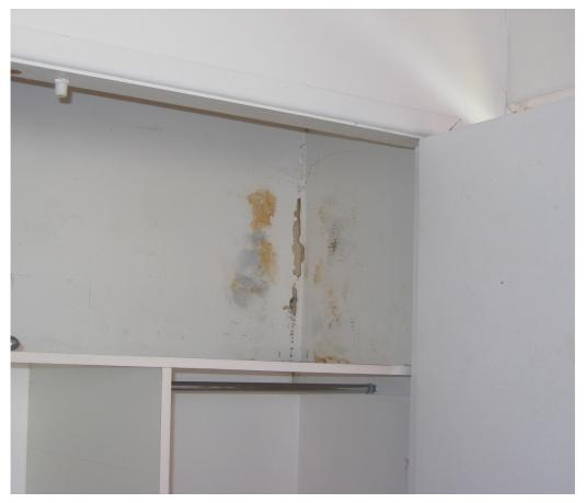
Same cupboard, but the other end and high. Very obvious damp stains but being high, a different source, probably from the roof. This house had a flat roof so it was impossible to access the roof space to investigate further.
