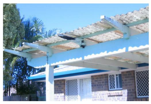
Rotting timber, no gutter, the roof is too flat and the fibreglass roofing is badly deteriorated, but even in this condition, it is still providing good shade to the back of the house. There is probably not much salvageable, so get a quote to replace it and add the cost to your budget.
